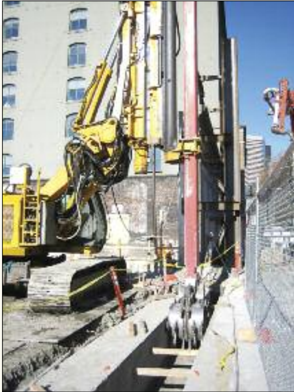
Figure 9 – Guide walls for initial alignment.
