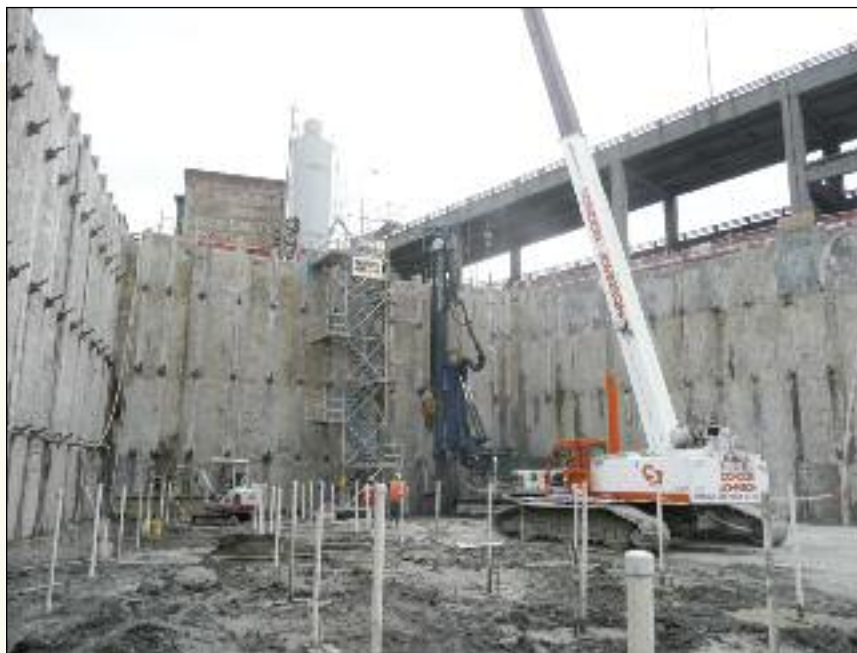
Figure 8 – Completed excavation and tiedown installation prior to placement of mat foundation
