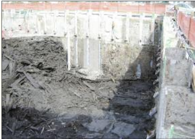
Figure 4 – Full extent of wood debris encountered during excavation and tiebeck installation
