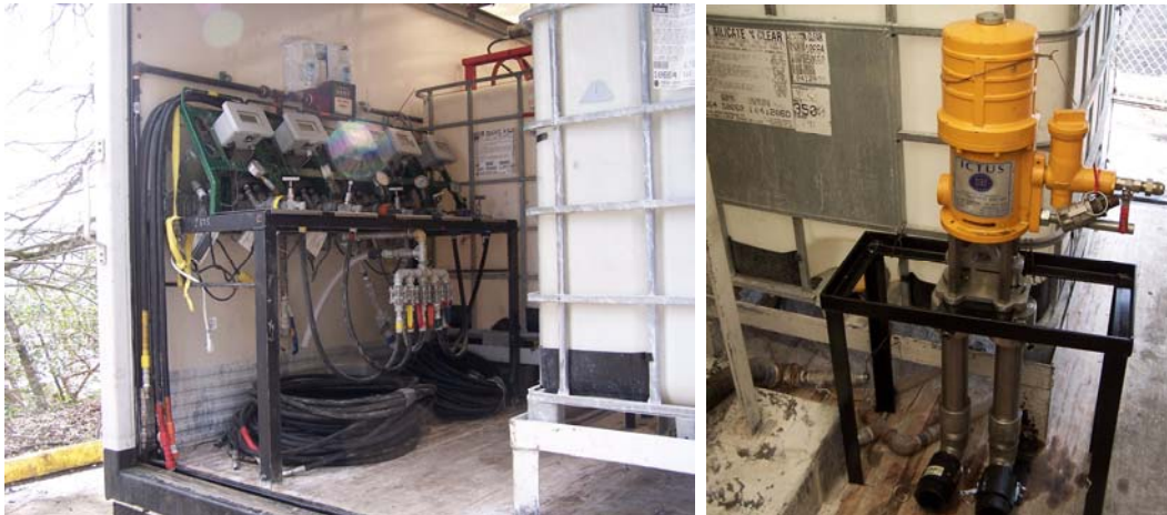
FIG. 6: Grout Truck and Dual Piston Pump
