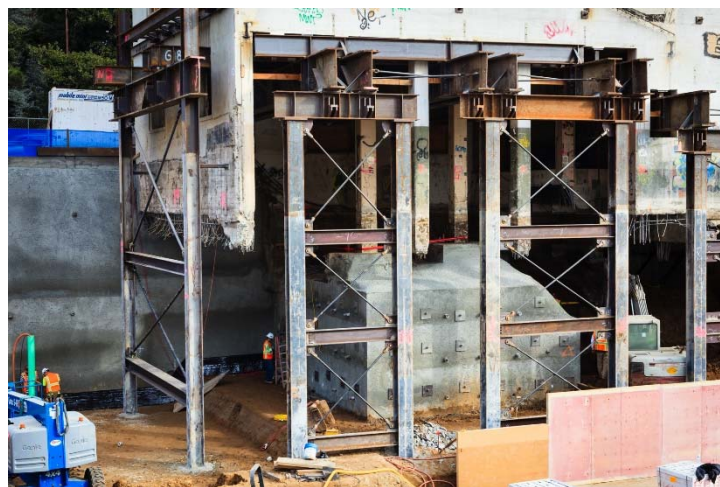
Figure 10. North End of Admin Block (Photo property of Alejandro Velarde)
