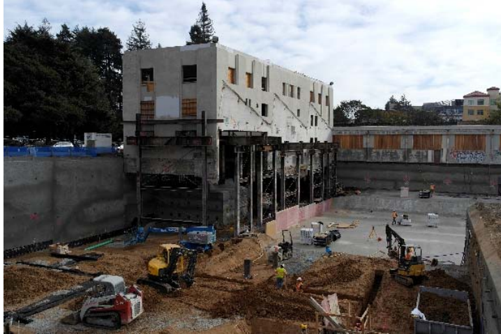
Figure 8. Admin Building Underpinning from Inside the Site (Photo by Degenkolb Engineers)
