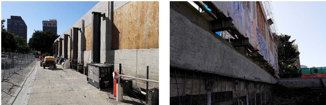
Figure 3 (left). Soldier Pile Extensions at South Wall
