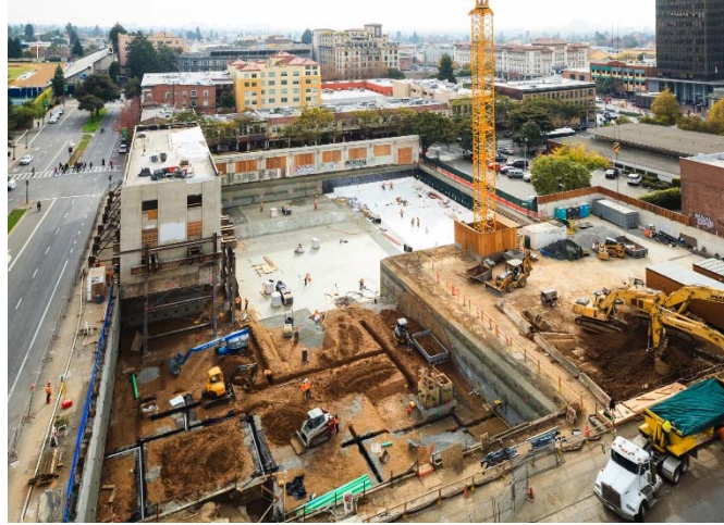
Figure 11. Completed Excavation (Photo property of Alejandro Velarde)
